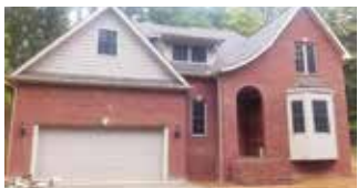
New Construction. 3 BR, 2.5 BA, large kitchen. (131142) $219,000 Call Shane 304-634-5993
