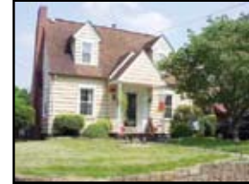
No Work Needed HW floors. Lots of recent additions. $110,000 #129714 Mike Ballard 304-416-9412
