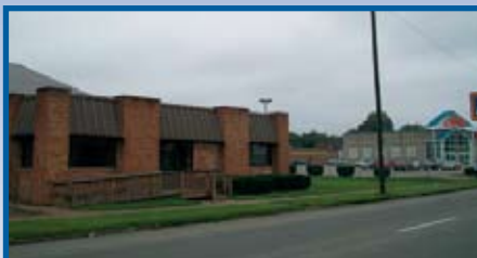
6,633 SQ. FT. in warehouse and 1,472 Sq. Ft. in office. Great visibility on busy street. (118106) $425,000 Call Barat 544-6080
