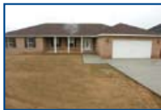
Applewood Rancher Brand New Home Big Rooms, Lots of Storage! $239,900
