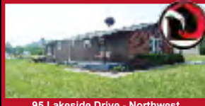
95 Lakeside Drive - Northwest
