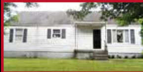
280 Haverhill OH Furnace Rd., FF
