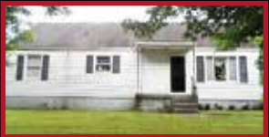
280 Haverhill OH Furnace Rd., FF
