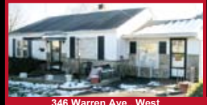
346 Warren Ave., West
