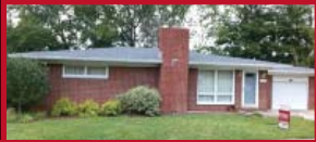
10127 High Street - Northwest
