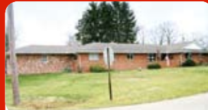
Wonderful 3 BR, 2 BA brick home. Spacious living room, master suite, heat pump, 3 car garage. $189,500
