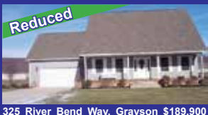
325 River Bend Way, Grayson $189,900 3 BR, 2 BA, 1.5 story. Well equipped kitchen w/appliances, MBR on main w/MBA featuring shower & whirlpool tub. Screened porch, garage plus more. Nancy Burchett 922-6263
