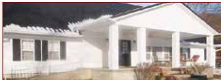
7729 Cannonsburg Rd - Recently renovated from top to bottom! The perfect country home awaits you with this 2,776+/- sq.ft. on 14.75+/- acres. This home has lg 4 BR (2 master suites) & 3 BA. Newer oak cabinetry & tile floor in kitchen. Original Oak flooring along w/newer beautiful laminate flooring. Fully fenced w/solar electric fencing around the entire perimeter of the property, plus newer stall barn. Almost all the land has been cleared. $225,000
