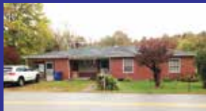
2003 Cannonsburg $62,000 3 BR, 2 BA, 1 acre, brick ranch. HW floors, newer roof, 2 wells on property. Could be really nice w/TLC. M280308 John Daniels 922-7633
