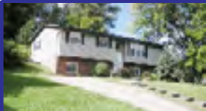
1902 North St. $69,900 2 BR, 1 BA double wide (bi-level) w/fin. bsmt foundation, new metal roof. HVAC - 3 yr old. Newer replacement windows + more. M410964 Brenda Burns 922-4052, Ed Cheek 465-0004
