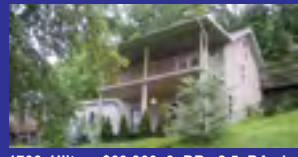
1706 Hilton $69,900 3 BR, 2.5 BA, lg remodeled 2 story. Newer roof, heat & air, windows, vinyl siding, flooring, light fixtures. Lg covered porches plus more. M241391 Brenda Burns 922-4052, Ed Cheek 465-0004
