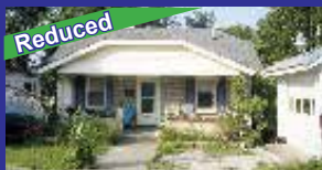
418 Laurel Ave. $62,900 2 BR, 2 BA, newer siding & windows, covered porch, det. garage, metal bldg. Some wood floors. Bsmt could be 3 rd BR. M401273 Brenda Burns 922-4052, Ed Cheek 465-0004
