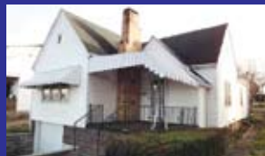
3230 Blackburn Ave. $69,500 2 BR, 1 BA cottage. Some HW floors. Fenced back yard w/alley parking. Laundry hookups in bsmt & main. FR could be 3 rd BR. M157666 Angela Coovert 571-6296
