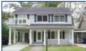
2614 Forest Ave. - 2 story Colonial style home w/4 BR, 2 BA, FR w/sliding doors leading to deck w/hot tub that remains w/the home. MBR features a balcony & walk-in closet. Lots of storage in the full size bsmt. Newer HVAC. This is an estate property & is being sold "As Is". $115,900 M140869 (PC)
