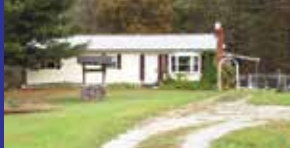
3265 St. Rt. 3307, Greenup $189,900 3 BR, 1.5 BA on 26+/- acres. Newer metal roof, HVAC & windows, lg metal bldg, barn, 2 car det. garage, inground pool. M276901 Denise Cumpton 694-3137
