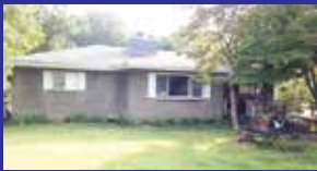
159 Robin Rd., Russell $119,900 3 BR, 1.5 BA ranch brick in walking distance of Russell schools. Unfin. bsmt that could be finished to make another BR & FR. M262664 Johnna McGuire 615-1927
