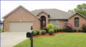
12907 Princland Heights Ct. $249,000 3 BR, 2.5 BA, 9 yr old ranch. Open floor plan & quality amenities. Screened porch, deck, stone frpl on patio. Much more. M254506 Missi Adkins 923-3129
