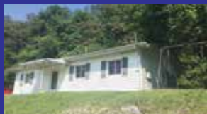
3261 Hickory St., Catlettsburg $35,900 3 BR, 1 BA, laminate flooring throughout, window AC, metal roof, det garage, private dead-end street. Laura Morris 606-923-6983
