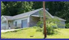
3001 Green Hill Dr., Flatwoods $129,000 3 BR, 1.5 BA custom built, one owner, constructed w/steel beams & open concept. Spacious FR, garage, carport & more. Bea Rice 606-831-9449
