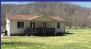
14 JR Junction, Hitches $64,500 3 BR, 1 BA ranch w/fenced back yard. Property goes back to creek. Furnished kitchen, back porch & deck. Libby Fugitt 606-571-6401
