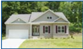
Russell - NEW CONSTRUCTION! Ready to move into this 3 BR, 2 BA home w/great room, eat-in kitchen, great master suite w/walk-in closet & whirlpool Jacuzzi tub. $179,900 #26431 (CJ)
